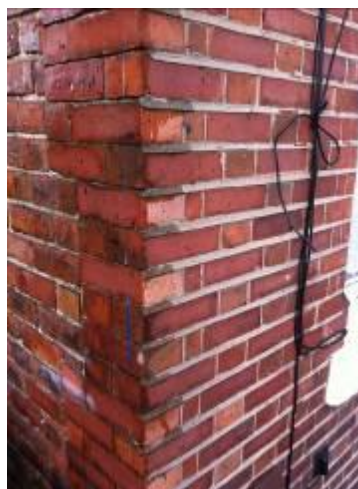
Hard cementitious ribbon pointing to front elevation
