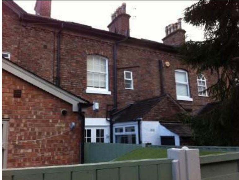
Surviving arched sash window to rear elevation, with modern outriggers in foreground
