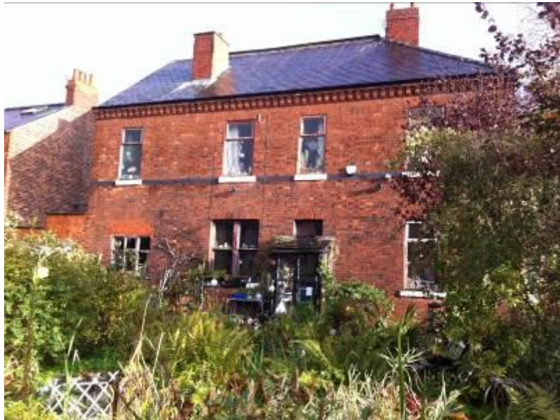
Modern casement windows flush with elevation, one bipartite sash window remaining to ground floor
